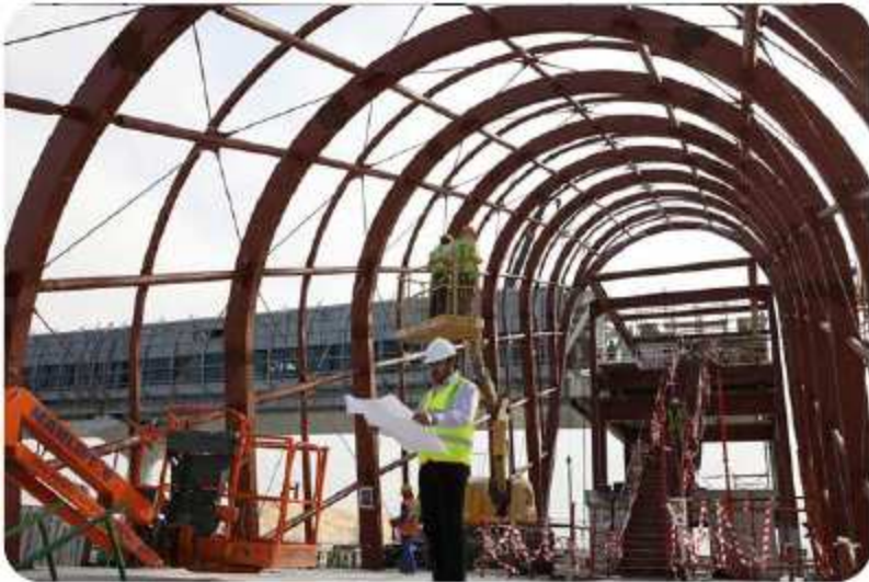
fabrication work STEEL HANGER
