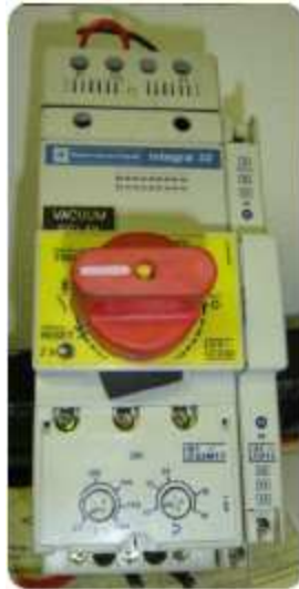
relay w base 230 telemechanique
