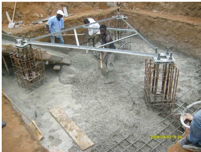
CIVIL WORK ALL TYPE
